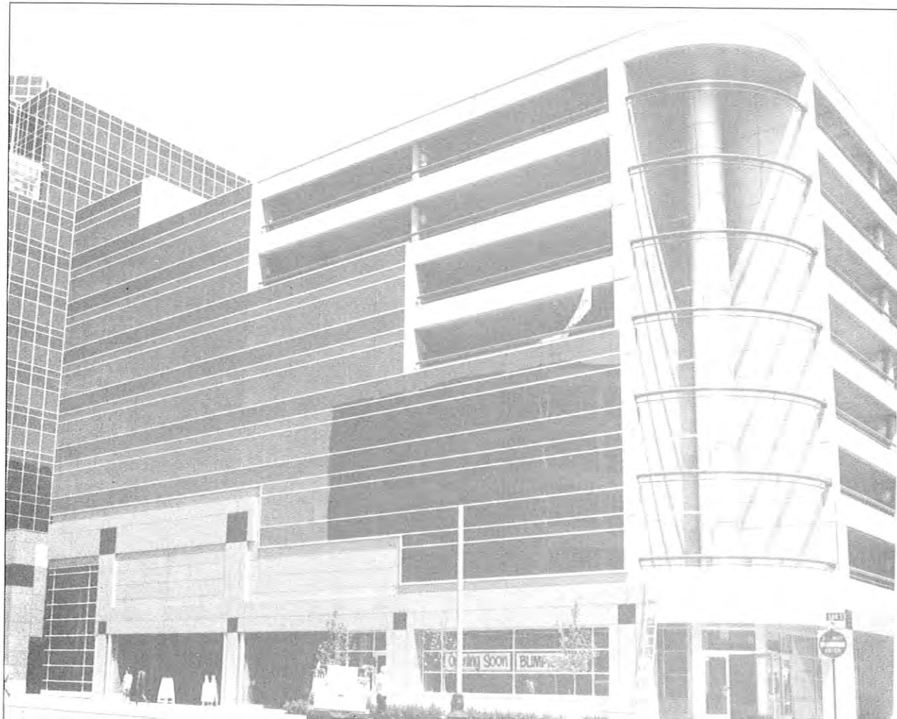
Broadway Centre Parking Structure, 1992
