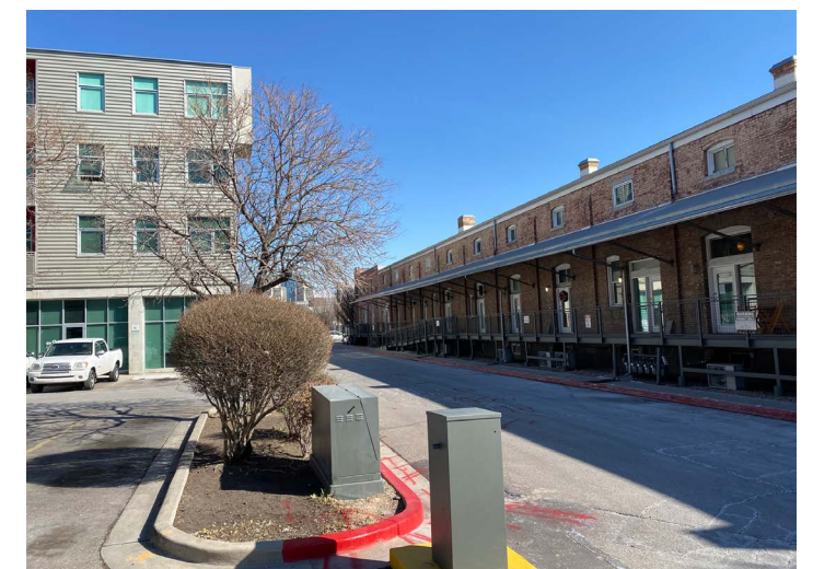
8 View of Eccles Avenue and the Artspace Bridge and City Center buildings looking east toward 500 West.
