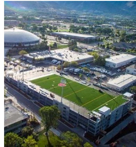
Figure 4.17: The Central Parking Garage at the University of Utah is a prime example of rooftop recreation on top of a parking structure.
