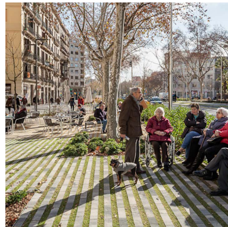
Figure 3.25: Permeable pavers can help with stormwater infiltration and reduction of urban heat island.
