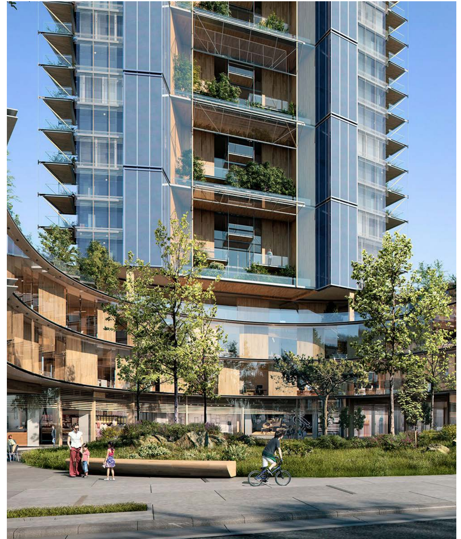
Figure 5.14: At 40 stories, Canada's Earth Tower will become the world's tallest hybrid wood tower, dramatically reducing the project's greenhouse gas emissions through carbon sequestration.
