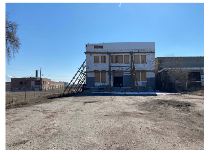
7 View of the existing Salt Lake Mattress Building looking south from 300 South.
