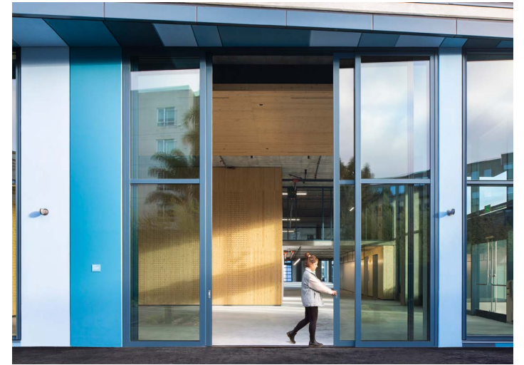
Figure 5.7: Sliding or roll up doors can facilitate the movement of people, equipment, and goods in and out of the ground floor.
