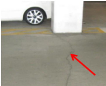
Figure 5: Medium Crack
