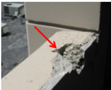
Figure 3: Concrete spall
