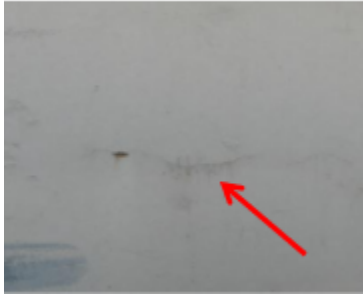
Figure 4: Fine crack
