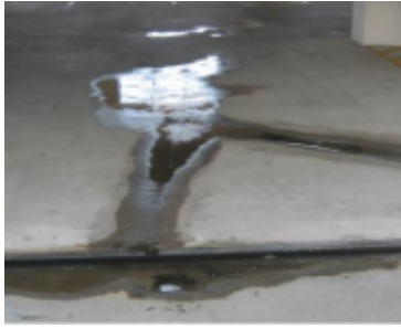
Figure 8: Ponding Water
