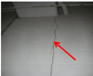
Figure 6: Wide crack
